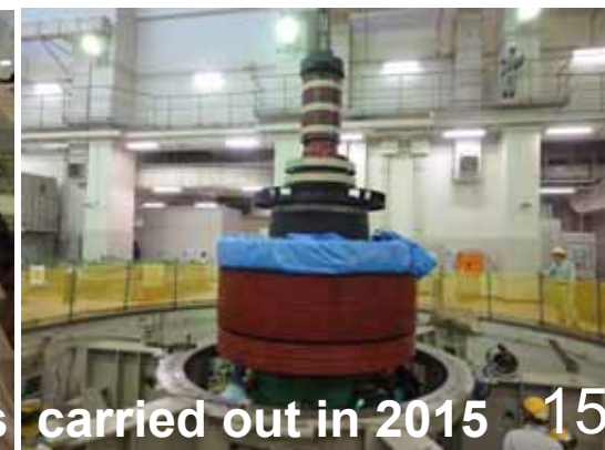
Overhaul of H-MG was
