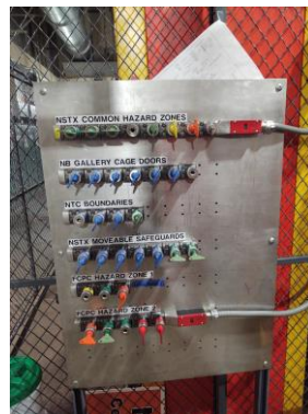
Trapped Key Exchange Blocks
