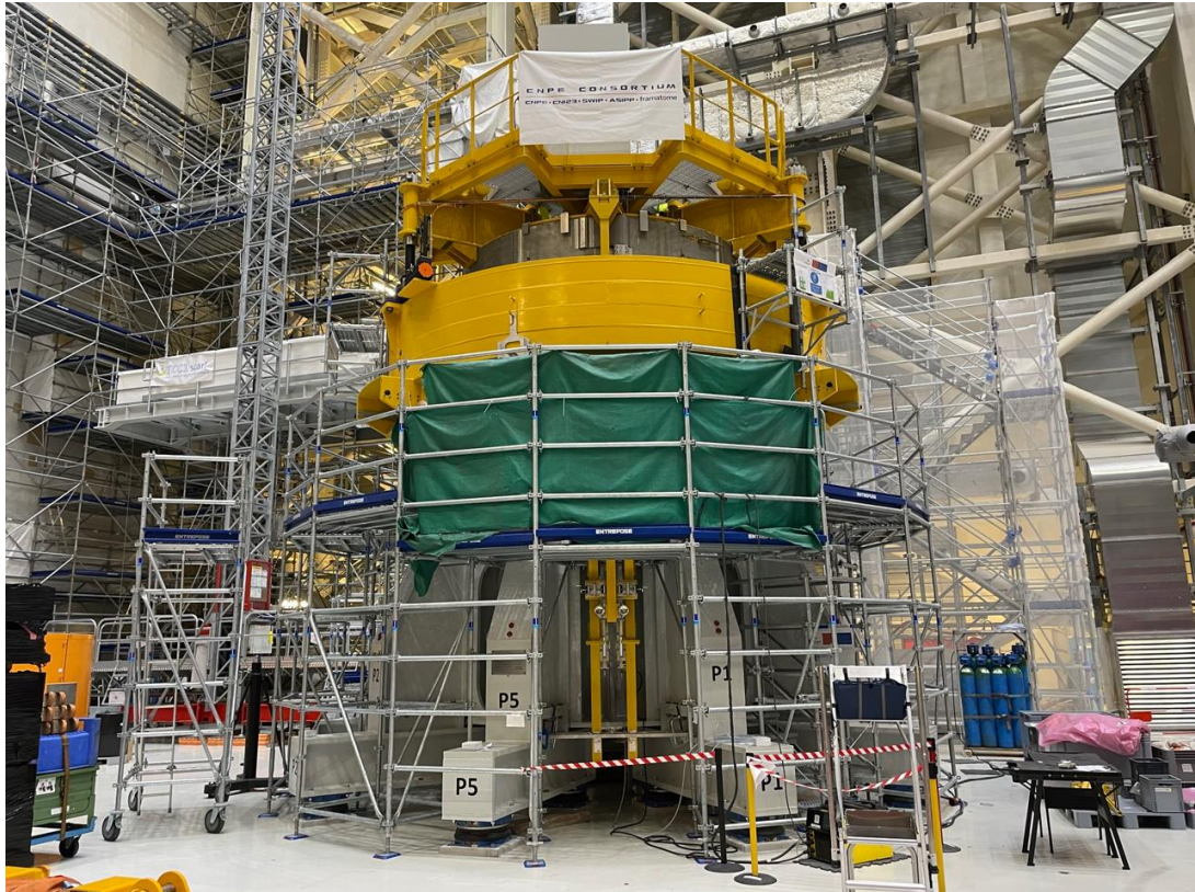
Module #1 installed on the base
