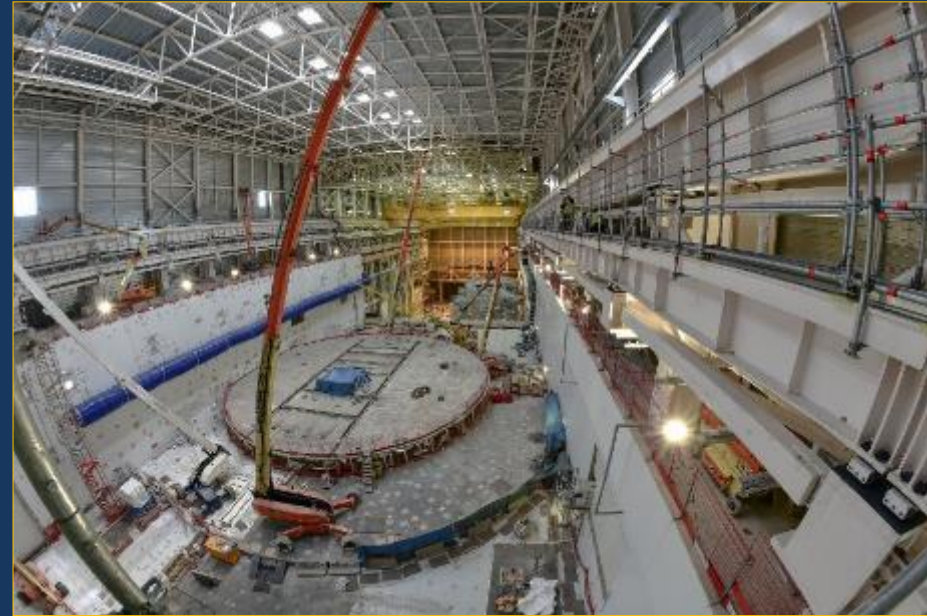
First crane access from Assembly Hall to Tokamak Building, 28 March 2020
