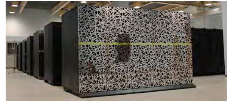
Helios system at Rokkasho site
